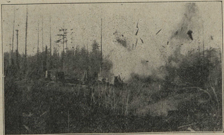
Blasting Big Stumps, Vancouver Island.
