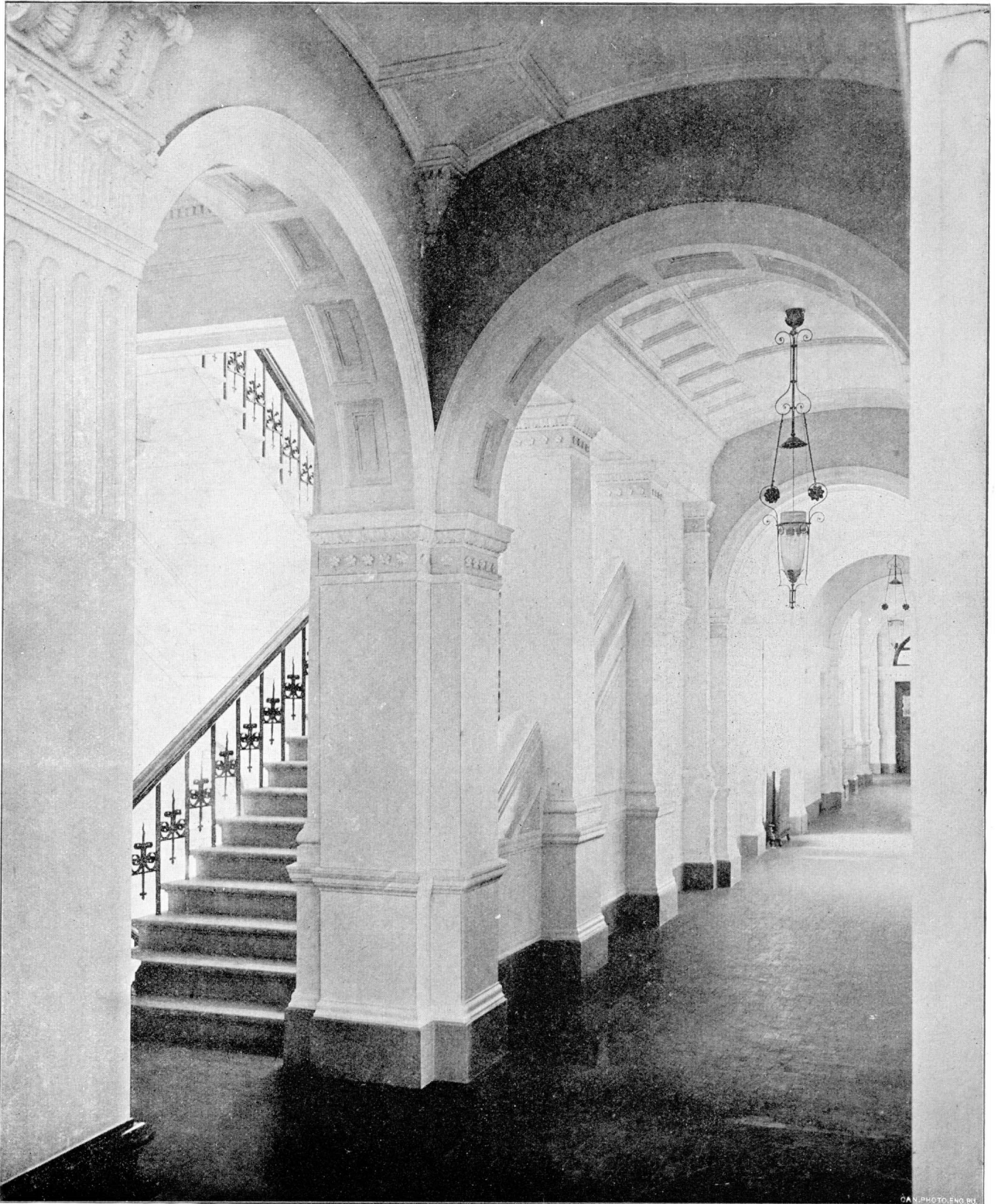
NEW LEGISLATIVE BUILDINGS, VICTORIA, B.C.—MAIN CORRIDOR, FIRST FLOOR, SHOWING SECTION OF STAIRWAY.
