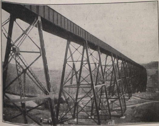
Fig. 1.—General View of Viaduct.
