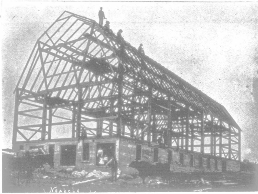
Barn of Archie Crozier, Beachburg, Ont. Size of wall, 45x120 ft. Wall, cistern and floor built with THOROLD CEMENT. The holes showing along the top of the wall are for ventilation.
