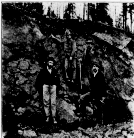
BODY OF ORE EXPOSED ON SNOWSHOE RAILWAY CUT.
