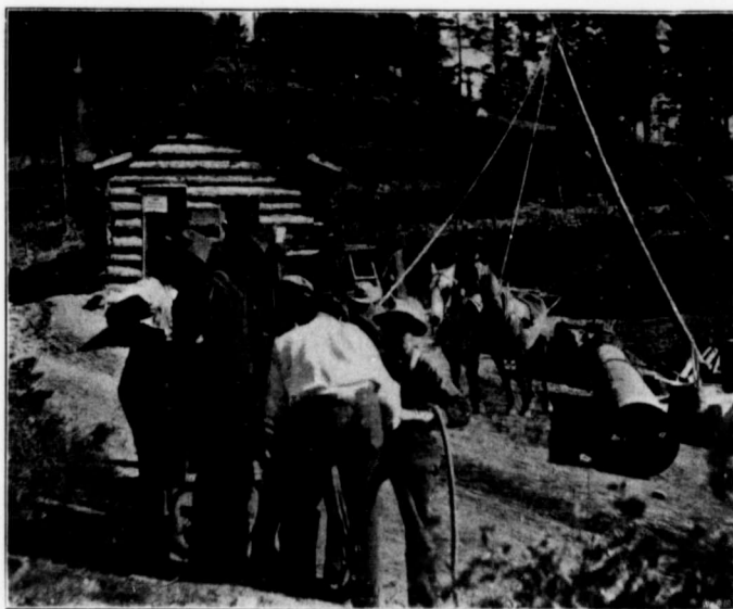
ERECTING SIXTY-FOOT SMOKESTACK FOR BOILER.
