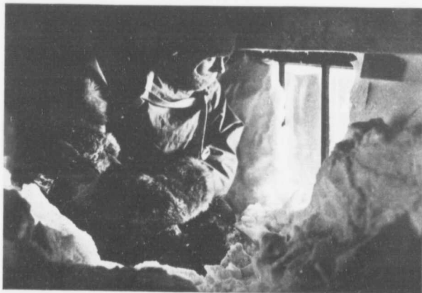
CLEARING DRIFT FROM WINDOW OF HUT AT CAPE ADARE
