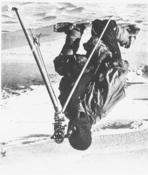
LIEUT. E. R. G. R. EVANS SCREENING WITH THE FOUR-INCH THEODOLITE WHICH WAS USED TO LOCATE THE SOUTH POLE.
