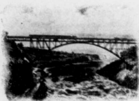
NEW STEEL-ARCH BRIDGE.
