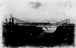
OLD SUSPENSION BRIDGE.
