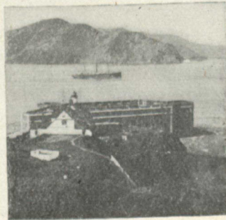
Fig. 26.—FORT POINT, AT THE GOLDEN GATE.
