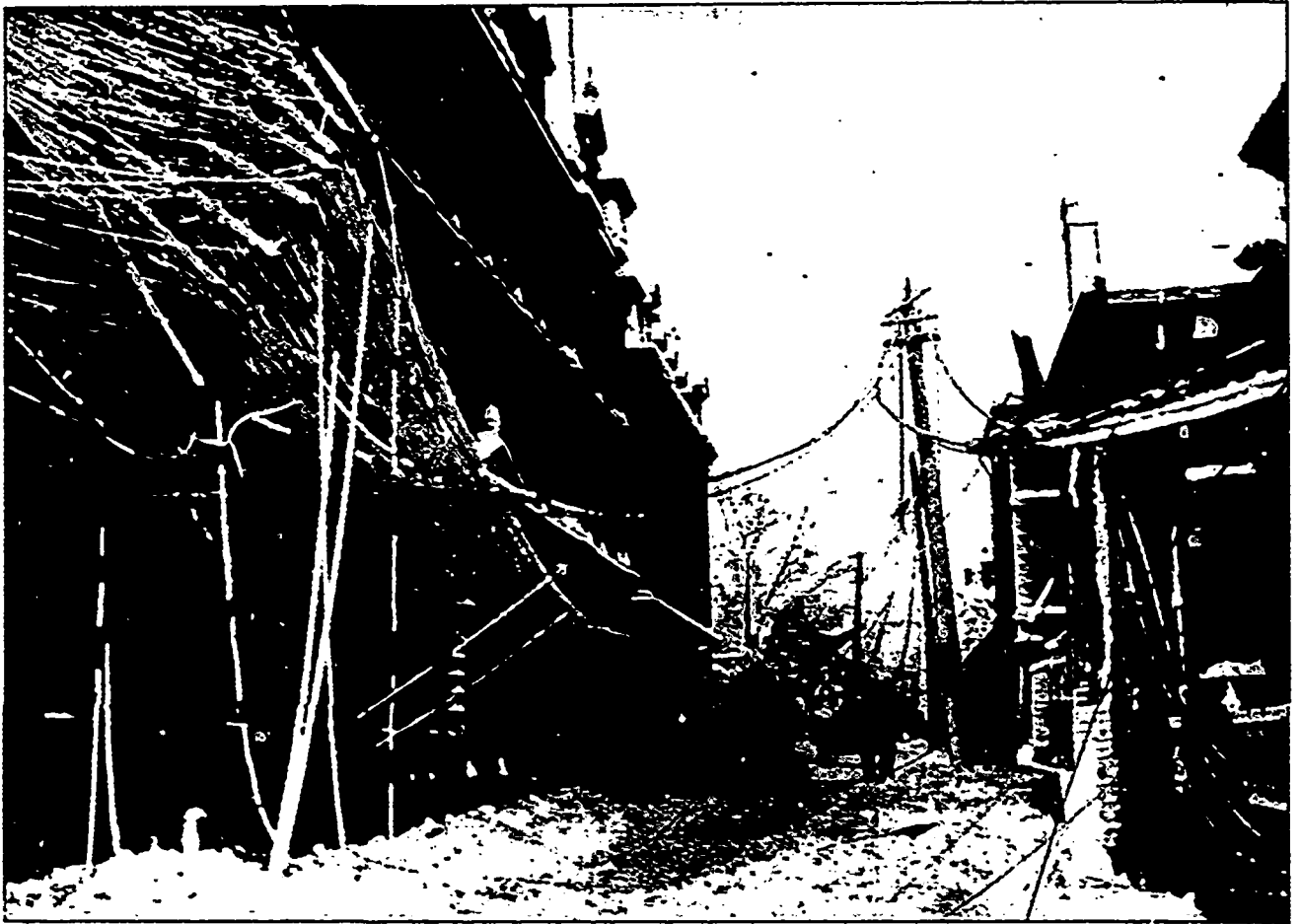
VIEW ON HUGHSON STREET, HAMILTON, SHOWING EFFECT OF THE RECENT SLEET STORM.
