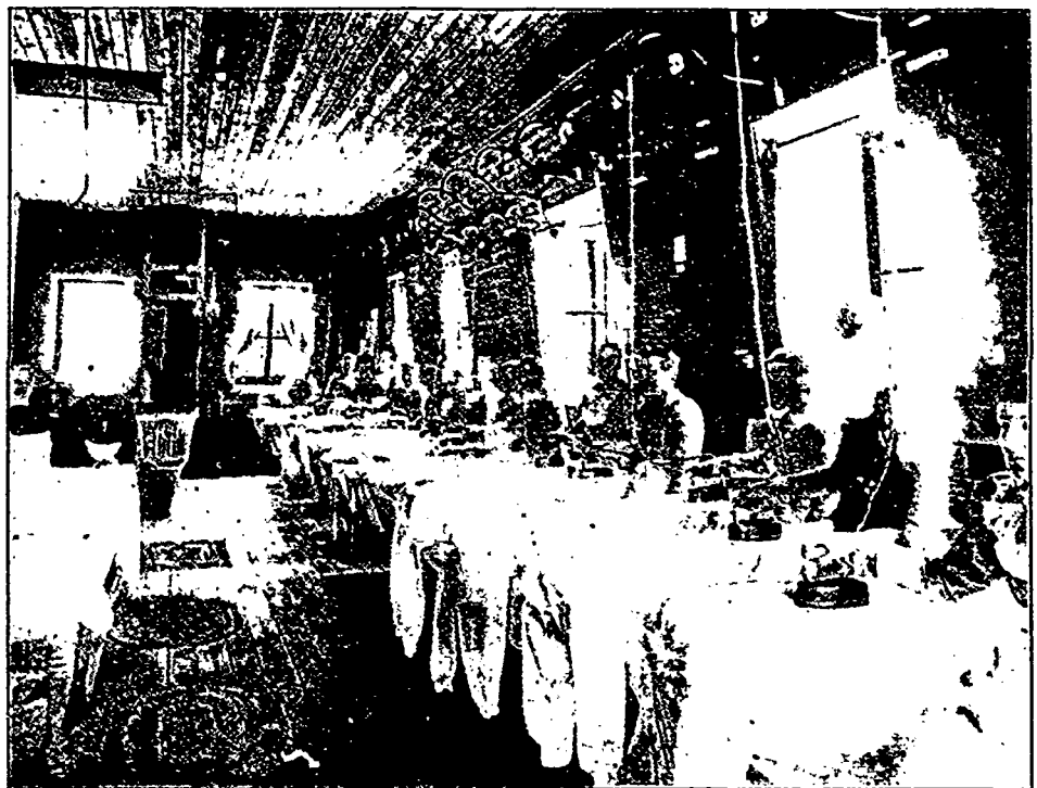
ELECTRIC PLANT AT BEAUPORT INSANE ASYLUM—IRONING ROOM IN LAUNDRY.
