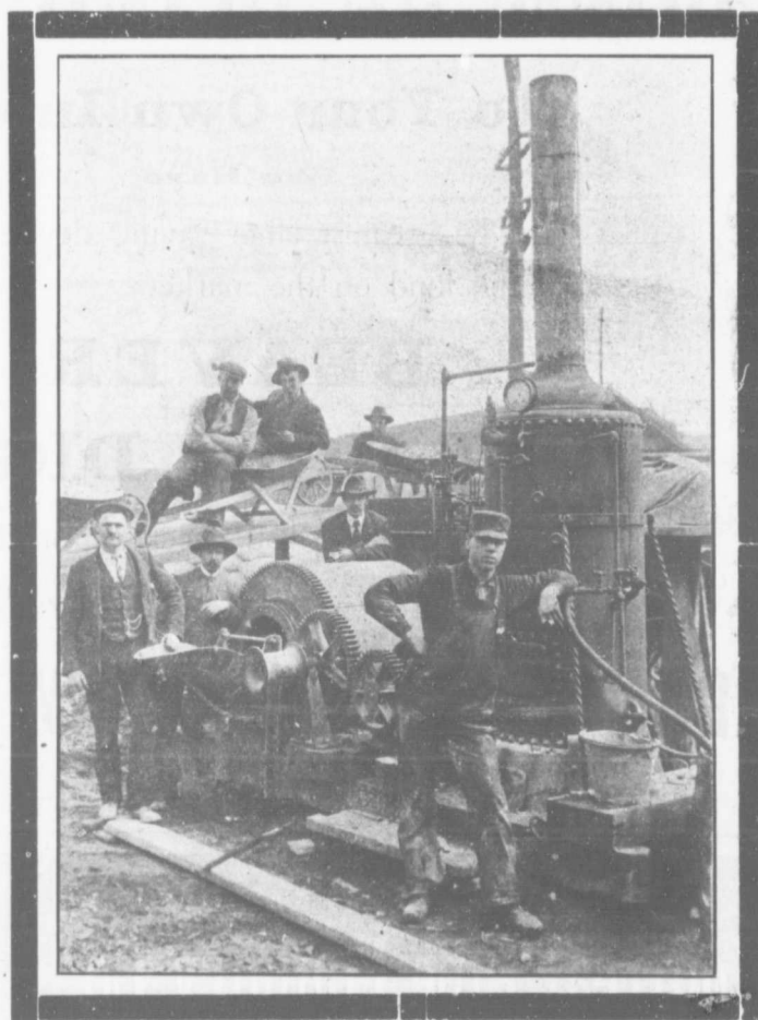
RANSOME CONCRETE MIXER OWNED BY R. A. ROGERS & CO., TORONTO AT PRESENT IN OPERATION AT THE CANADA FOUNDRY CO., TORONTO
