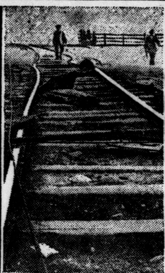
PICTURE on the left shows ruins of a convent at Haileybury, where the pupils were forced to stand waist deep in the waters of the lake to escape death by fire. The picture on the right shows railway tracks at Englehart warped by the intense heat. The T. and N. O. depot there was completely destroyed.
