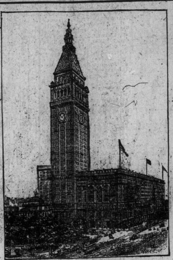
HOME OFFICE BUILDING. The largest Office Building in the world, Madison Ave., 4th Ave., 23d and 24th Sts., New York City
