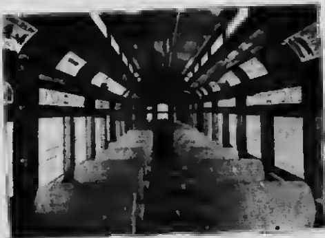
INTERIOR OF CARS USED IN INTER-URBAN SERVICE
