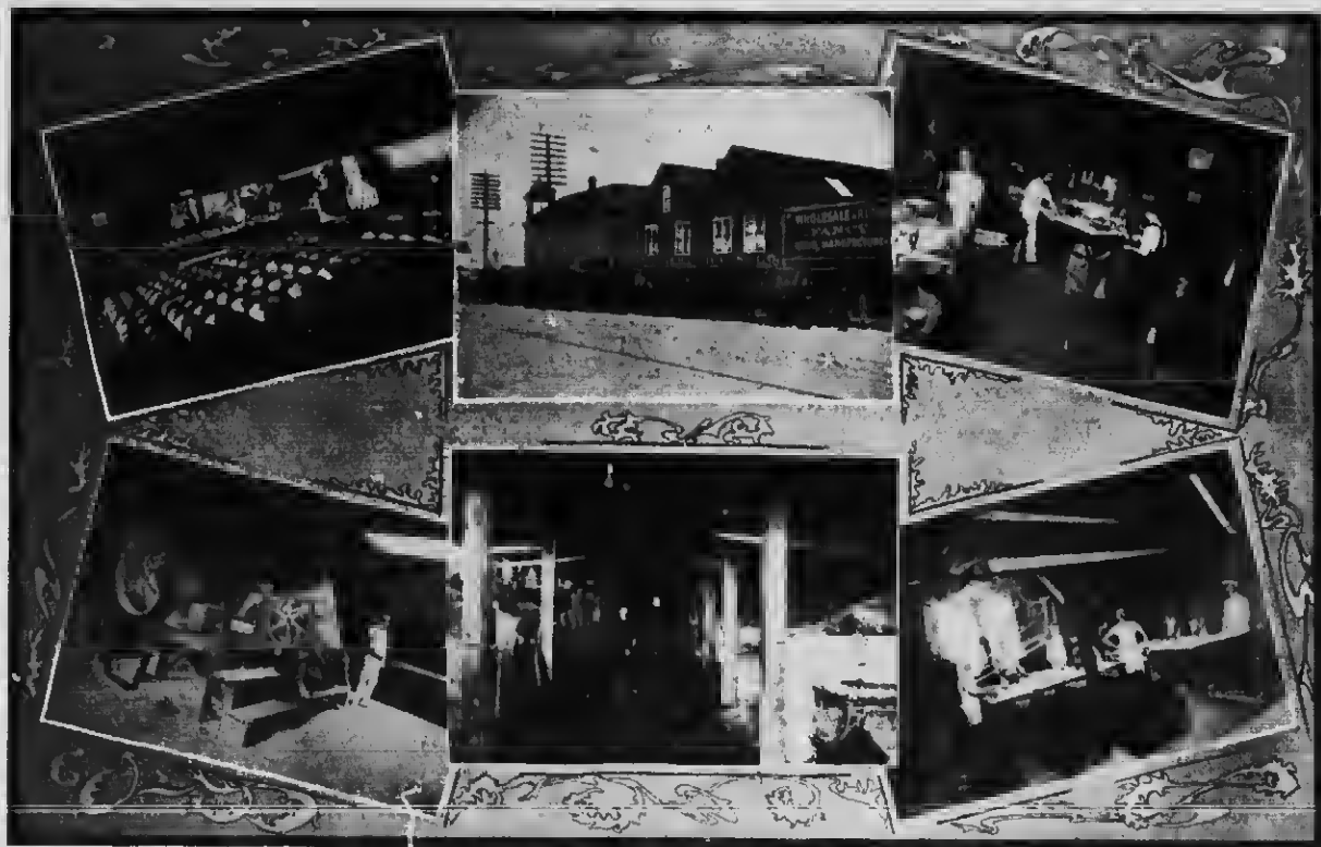
ILLUSTRATIONS OF THE MODERNLY EQUIPPED BAKERY OF HANBURY, EVANS & COMPANY 241 WESTMINSTER AVENUE
