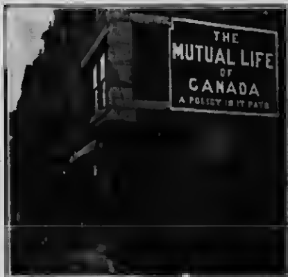
OFFICES OF THE MUTUAL LIFE OF CANADA FEE BLOCK, 570 GRANVILLE STREET
