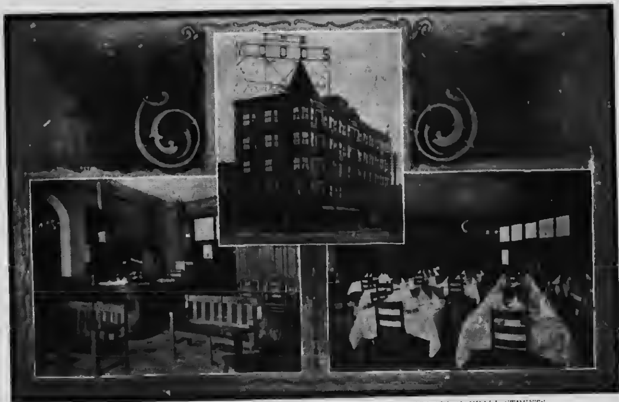
EXTERIOR, LOBBY AND DINING ROOM, WOODS HOTEL, CORNER HASTINGS AND CARRALL STREETS
