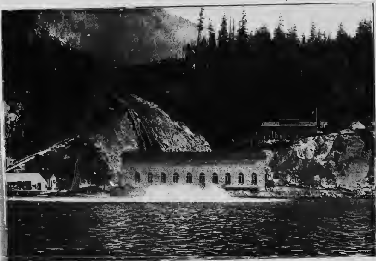
BRITISH COLUMBIA ELECTRIC RAILWAY COMPANY'S WATER POWER PLANT AT LAKE BUNTZEN
