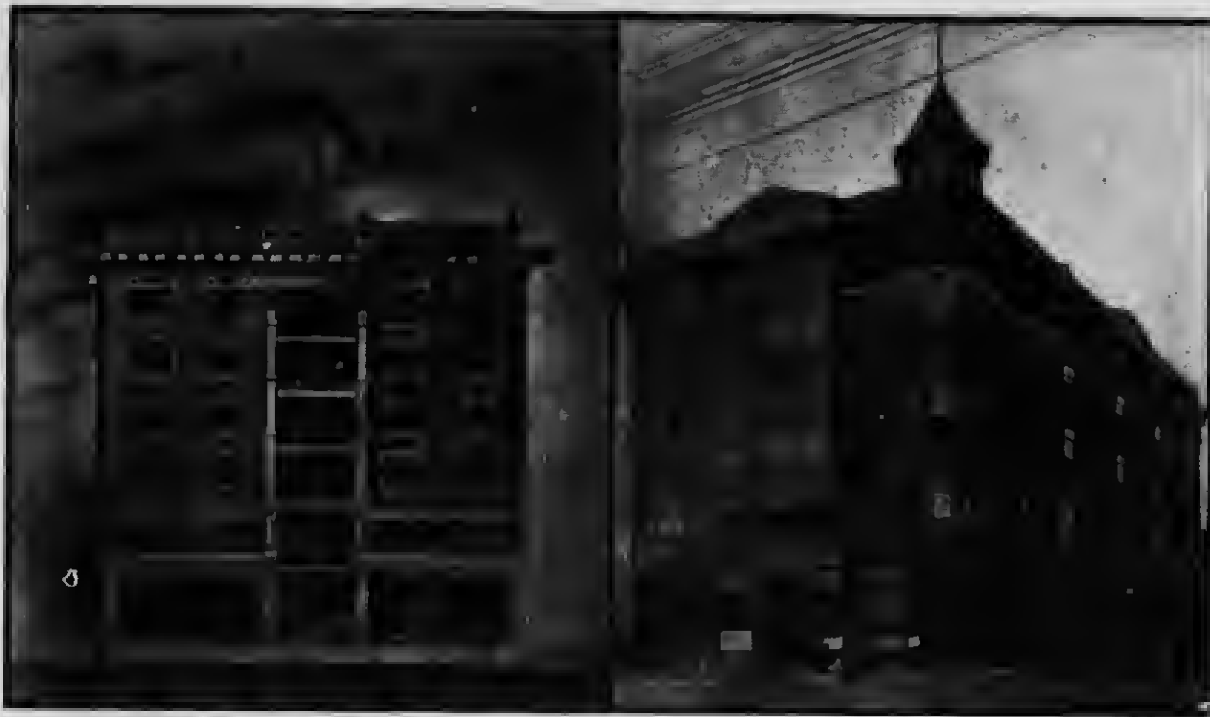
These buildings are owned by Granville Land & Loan Company, Limited, of which R. D. Rolison & Son are representatives
