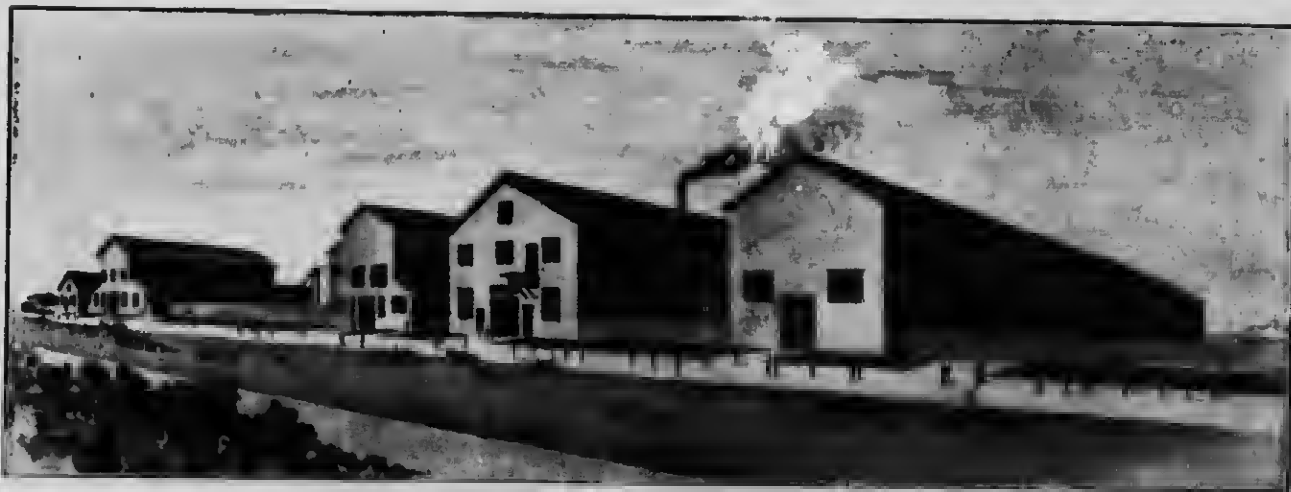
VANCOUVER ENGINEERING WORKS, SIXTH AVENUE AND BRIDGE STREET
