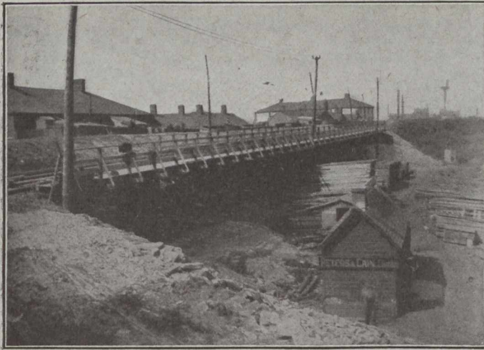
Fig. 7.—Sidehill Trestle. Old Fort Buildings in Rear. No buildings of the Old Fort were altered, the only disturbances were two cuts through the earth parapet, one of which is shown at the far end of the trestle.
