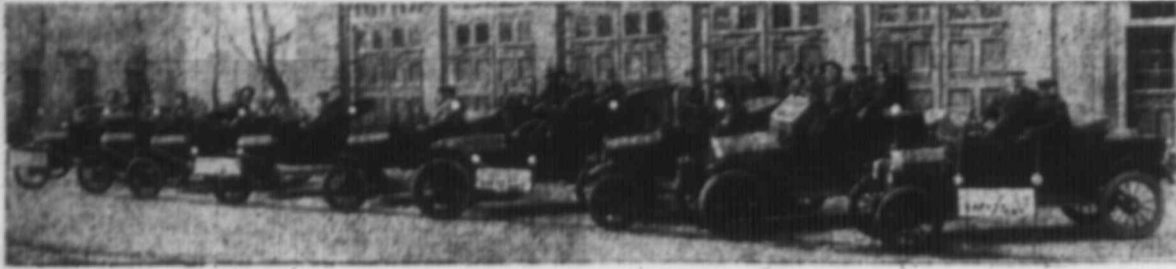
One of Our Installing Divisions
