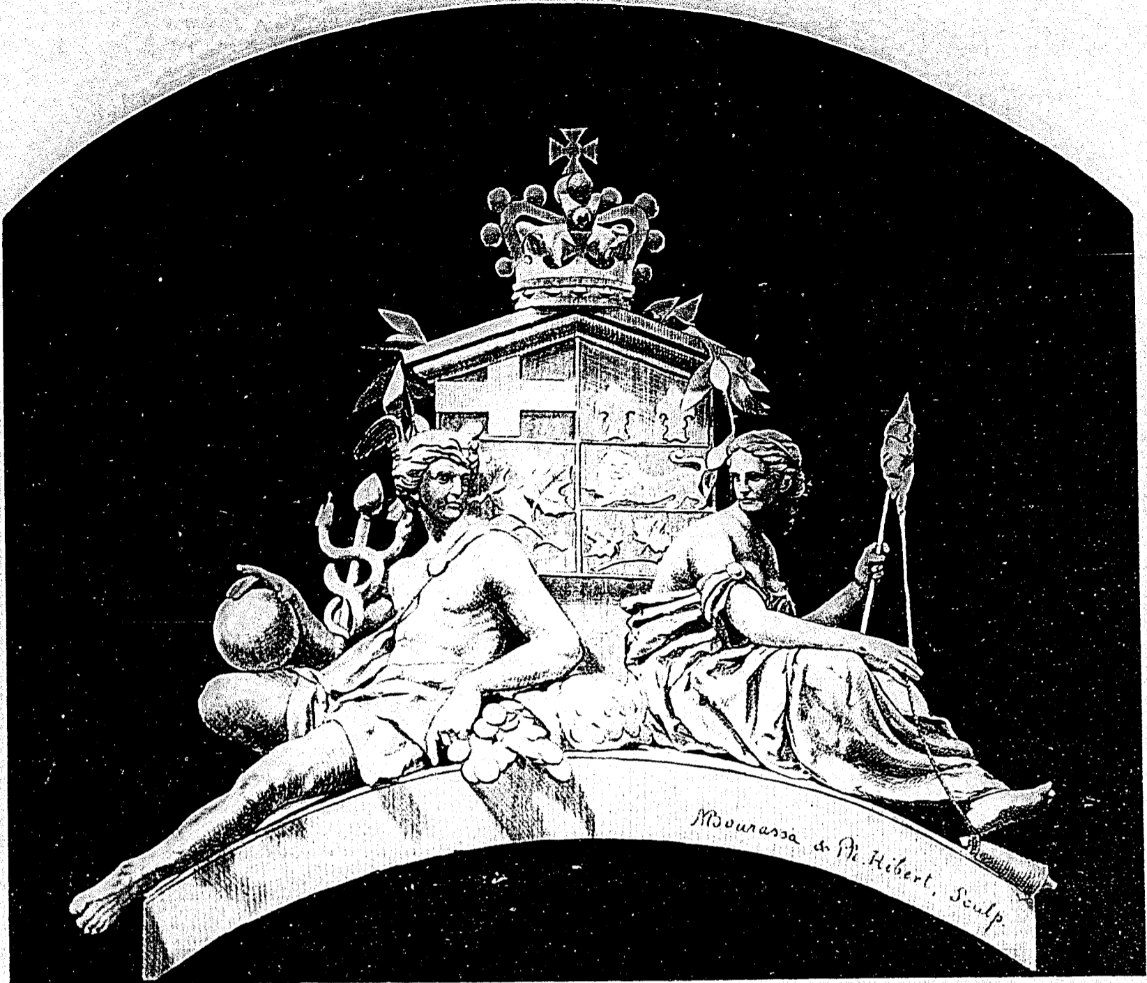
MONTREAL :—GROUP, REPRESENTING COMMERCE AND INDUSTRY, ERECTED ABOVE THE PEDIMENT OF THE NEW POST OFFICE.
