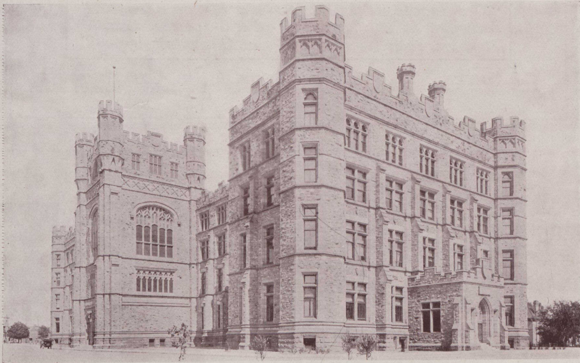
THE PRESENT PARLIAMENT BUILDING—THE HOME OF RECONSTRUCTION
