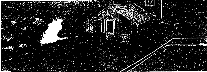
GARAGE AND GREENHOUSE, ERECTED FOR MR. J. D. CHAPLIN, ST. CATHARINES, ONT., BY LORD & BURNHAM CO., LTD. BECAUSE OF ITS COMPACTNESS AND ECONOMY IT PROVES A GOOD COMBINATION. HEATING OF BOTH IS ACCOMPLISHED BY THE USE OF ONE BOILER, SITUATED UNDER THE GREENHOUSE.
