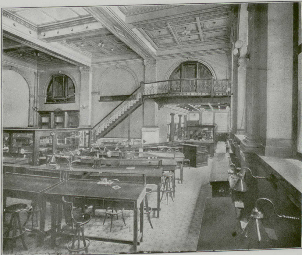
MAIN OFFICE, LOOKING TOWARD ENTRANCE.
