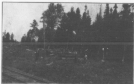
FIG. 13 Fire Hazard in Algonquin Park, Ontario, reduced through the disposal of inflammable material along Grand Trunk right of way and land immediately adjacent.
