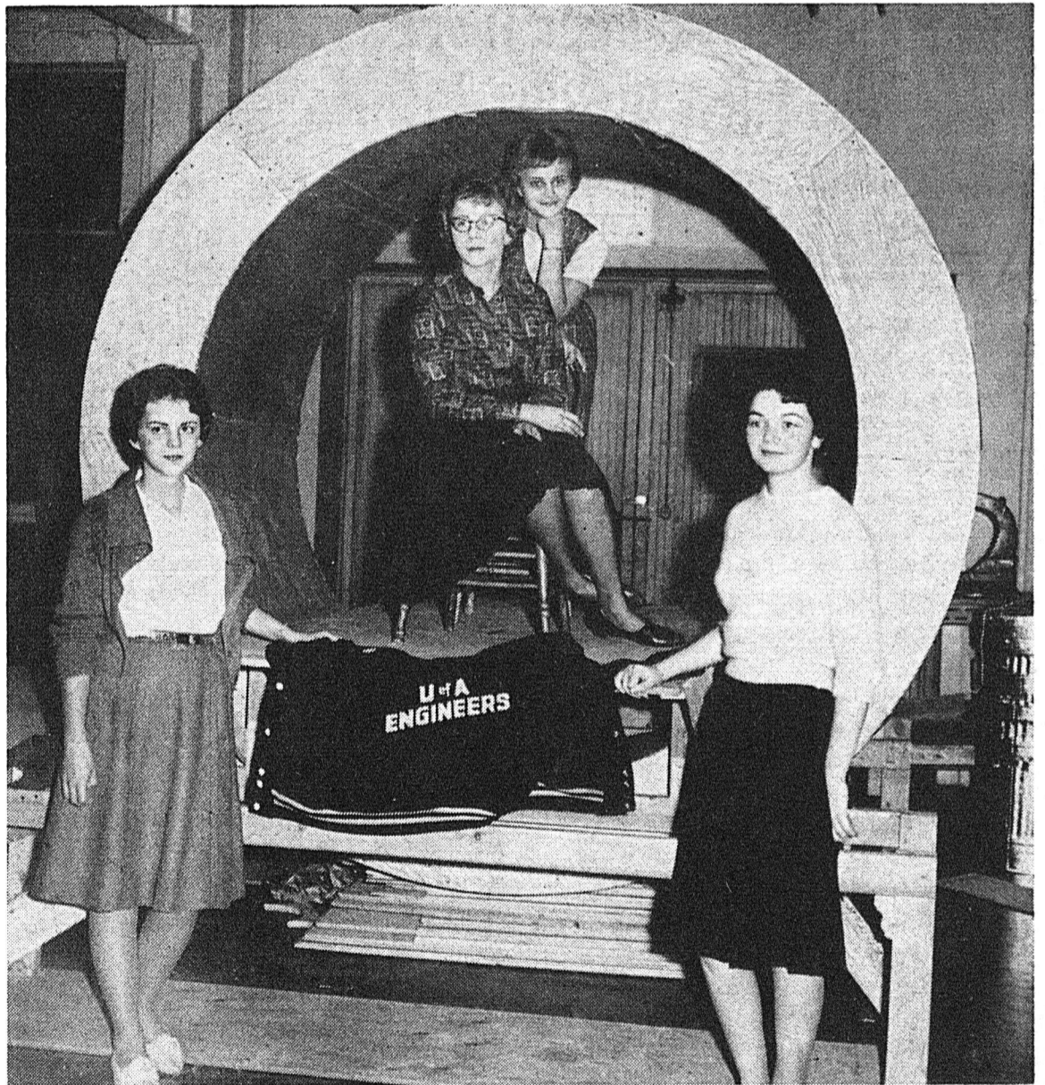
WONDERING WHERE THE BOYS ARE, four wandering Gateway girls investigate the ESS's float for Saturday's Homecoming parade. The float, now under construction in an engineering laboratory, consists of a large
