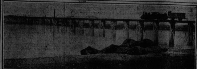
The bridge is about a mile long, and is to be replaced by a permanent masonry and steel bridge to cost \$3,000,000, and requiring three years to complete.
