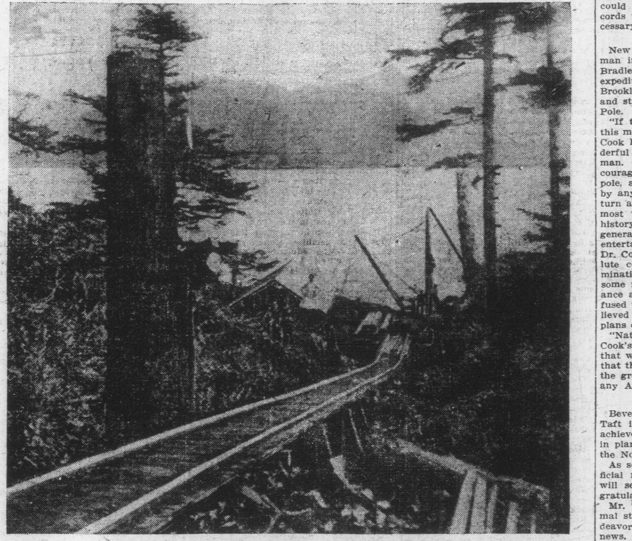
ENTRANCE ISLAND LIGHT, QUATSINO SOUND. The view is from Light House site, looking down the tramway to the water. At the bottom of the tramway is fixed a large derrick which picks up the stores and material from the boats just outside the breakers and lands them on the tramway. The work is under the charge of Thomas Tubman.
