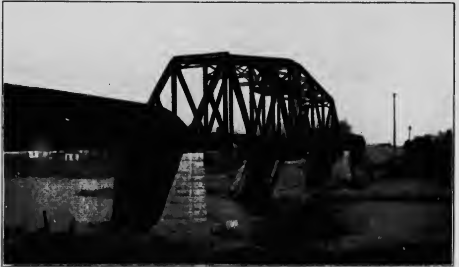
Assiniboine River, Headingly. Meter section at Bridge.
