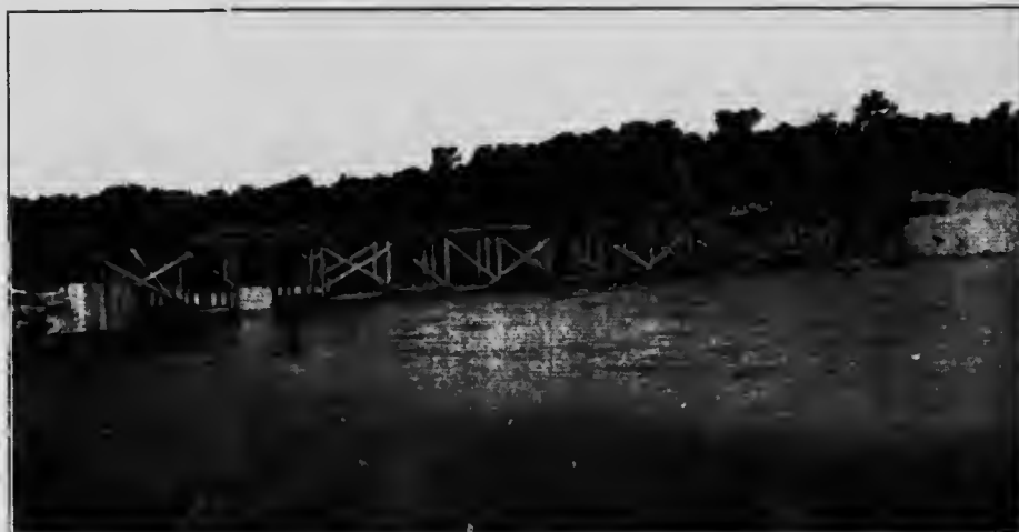
Fairford River at Fairford. Meter Section at Bridge, 1912.
