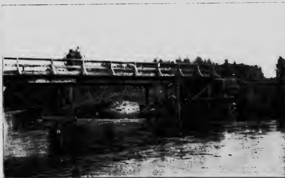
Brokenhead River, Sinnot. Bridge, showing gauge.
