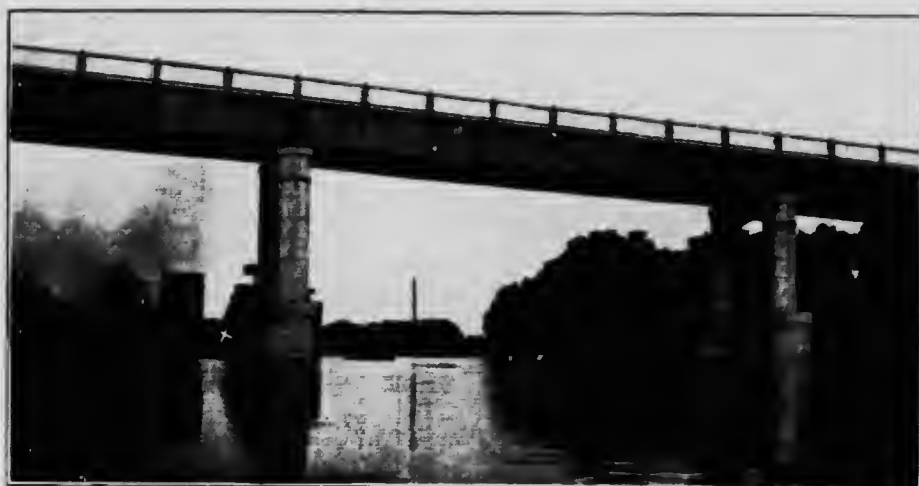
Assiniboine River, Brandon. Gauge at Bridge.
