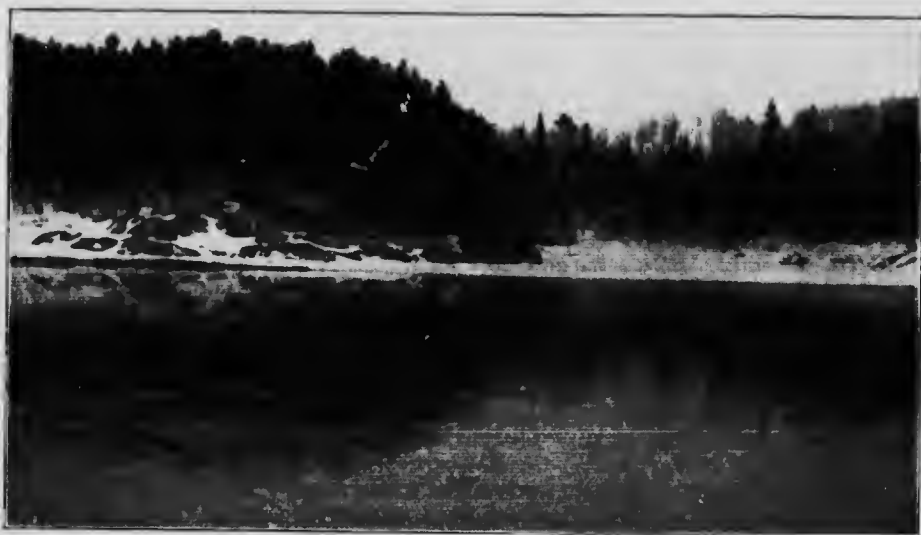
Winnipeg River, Slave Falls. Metering section.
