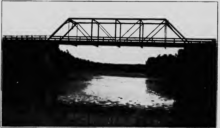
Souris River, Wawanesa. Meter section at Bridge.
