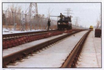
The LRT system connects Toronto's extensive transit network with the outlying Scarborough Town Centre and Civic Centre. Here, Philips' cable is pulled between Midland and Kennedy Stations.
