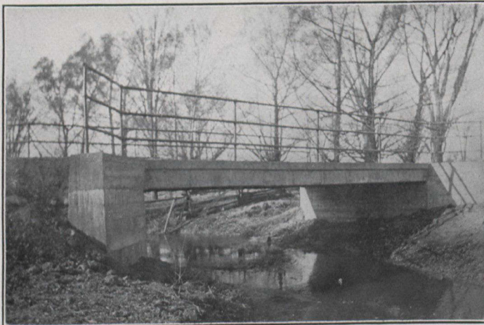
Concrete Bridge near Hornby, Ont., of 30-foot span. The bridge floor is reinforced with four 12-inch "I" beams 30 feet long. Net cost less than $900.
