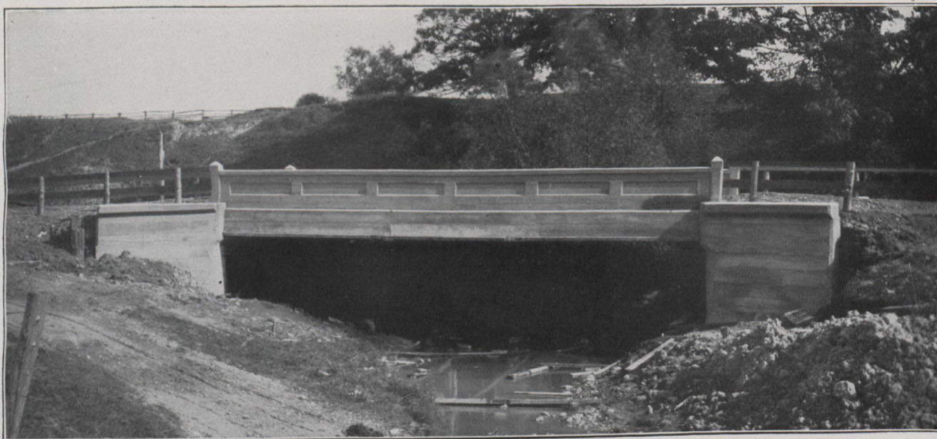
A 40-foot Beam Span, Mapleton, Ont.
