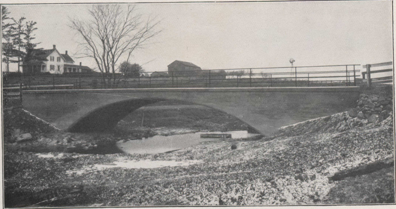
A 50-foot Arch Bridge at Buttonville, Ont., built at a cost of $2,400.
