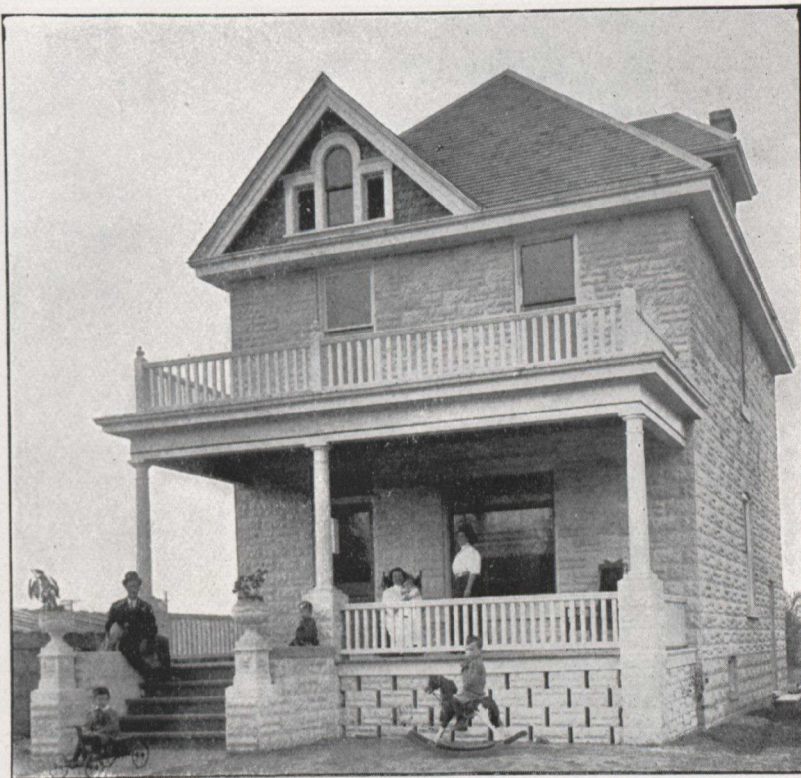
Concrete Block Residence of Mr. W. J. Howlett, London, Ont.
