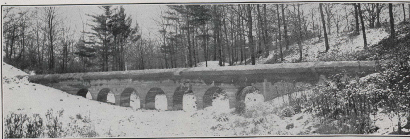
Concrete Viaduct, built by the City of Toronto, for carrying sewer pipe over Sunnyside Avenue Ravine.
