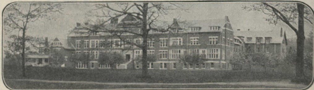
NEW BUILDINGS NOW BEING ERECTED
