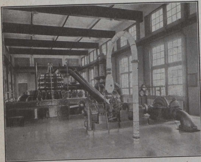
Another View of Pump-house, Showing Worthington Vertical Pump and De Laval Auxiliary Pump.
