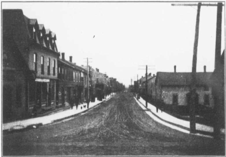
QUEEN STREET—LOOKING WEST FROM JOHNSTON'S CORNER.
