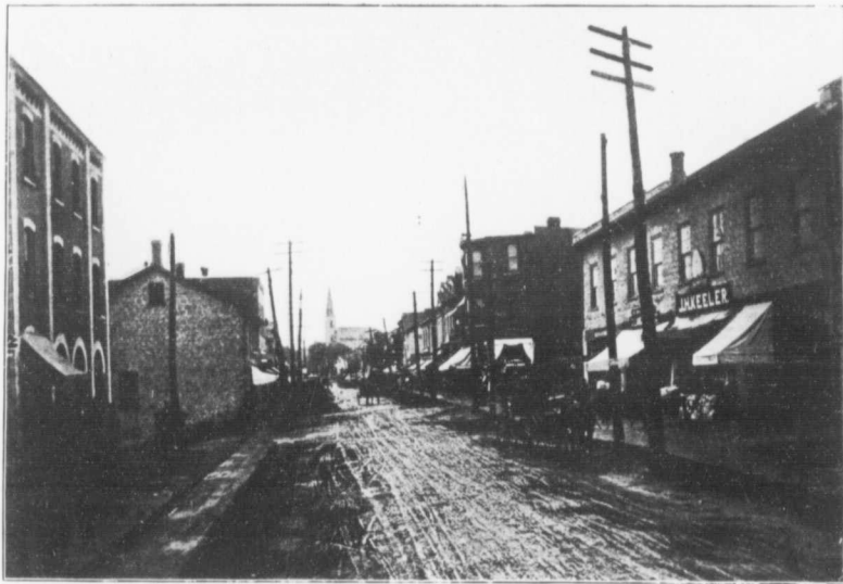
QUEEN STREET, BEFORE THE PAVEMENTS WERE LAID.
