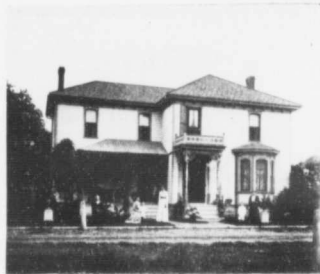
RESIDENCE OF W. B. VANDYKE, GRIMSBY.
