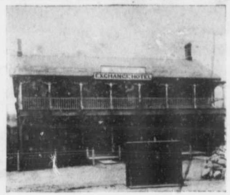
EXCHANGE HOTEL, STONEY CREEK.
