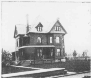
RESIDENCE OF GEORGE RILETT, WINONA.
