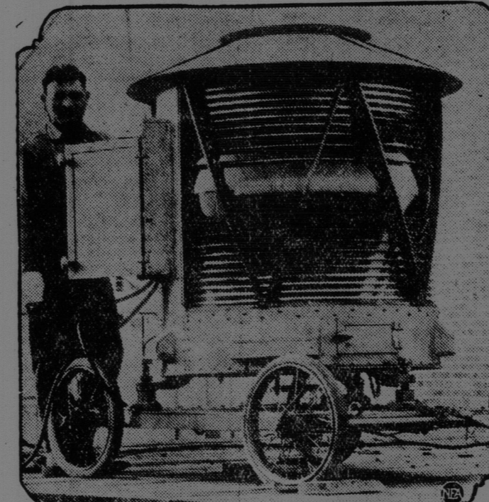
The most powerful lights in the world are being installed on all the air mail fields from New York to San Francisco. The lamps are a special 500,000,000 candle power B. B. field flood light, and their projected light covers an area of half a mile. You can read a newspaper two to three miles from it, and from the air it is visible for 75 miles.
