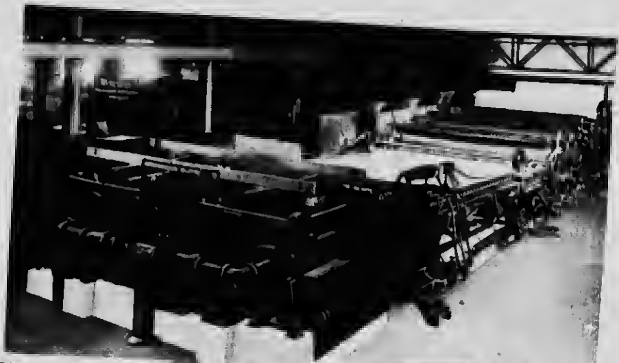
Wet End showing Screens, Wire and Presses
