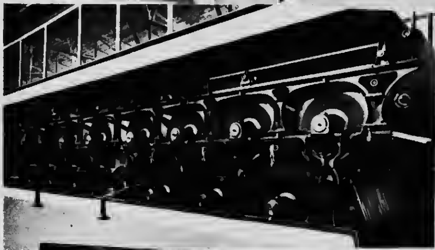
Section of Steam Heated Dryers
