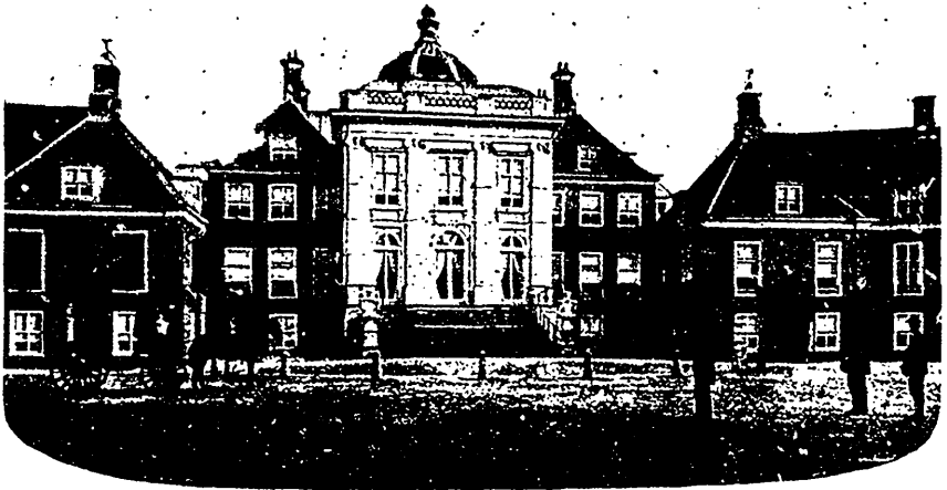
THE "HOUSE IN THE WOOD"—REAR VIEW.
