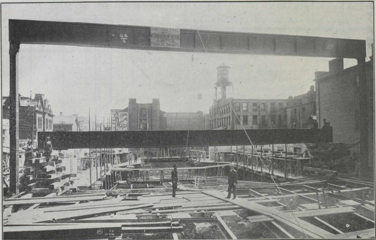
Balcony and Gallery Girders as Erected.
