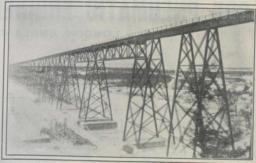
CAP ROUGE VIADUCT, NATIONAL TRANSCONTINENTAL RAILWAY.
