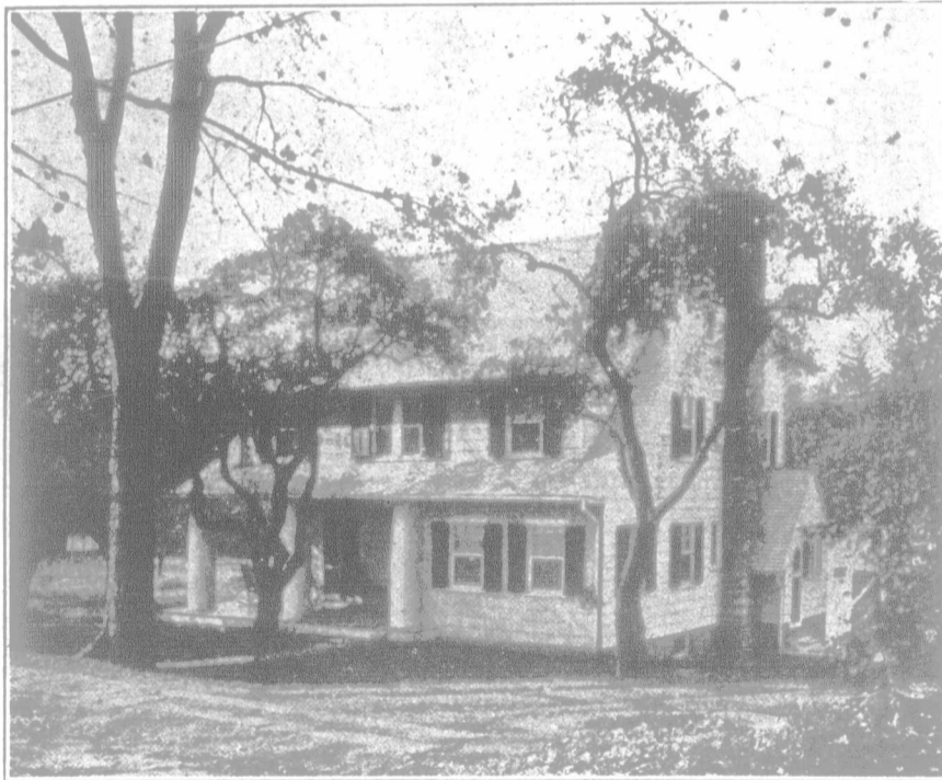
The Chimney May Be Built Outside.
