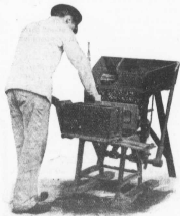
Opening doors. Block ready to be removed.
