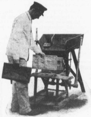
Changing face-plates. When machine is open face-plate is vertical, but is on the bottom when block is being made.
