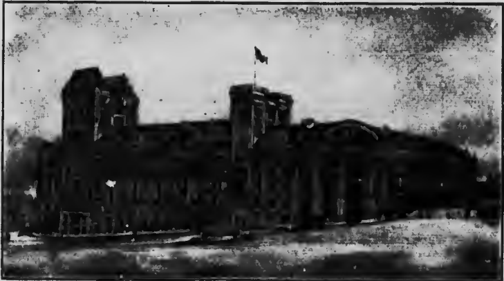
Canadian Pacific Railway Windsor Street Station.
