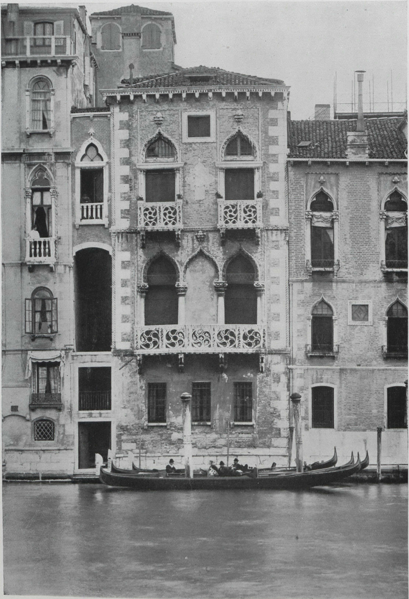
The Contarini-Fasan, Venice, built during the fourteenth century. This palace, which is often shown as the house of Desdemona, is one of the most exquisite of small Gothic structures in Venice, and is the only structure in that city that has traceried balconies.
