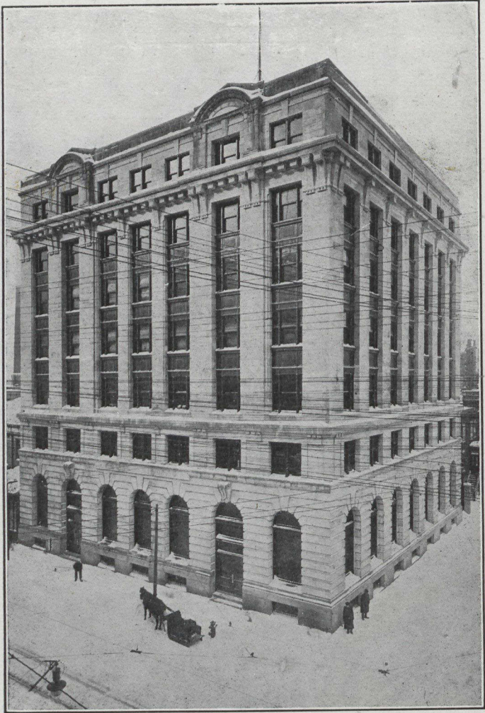
Montreal Light, Heat & Power Building
