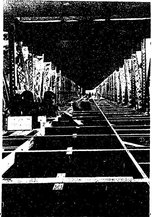
St. Andrew's Rapids Dam, showing the unobstructed working floor between trusses "A" and "B" and the highway floor beams overhead. H. E. Vautelet, Consulting Engineer.
