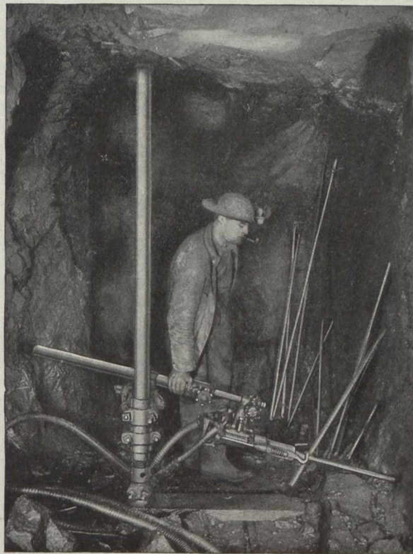
Putting in a "lifter" with the drill under the feed piston.
