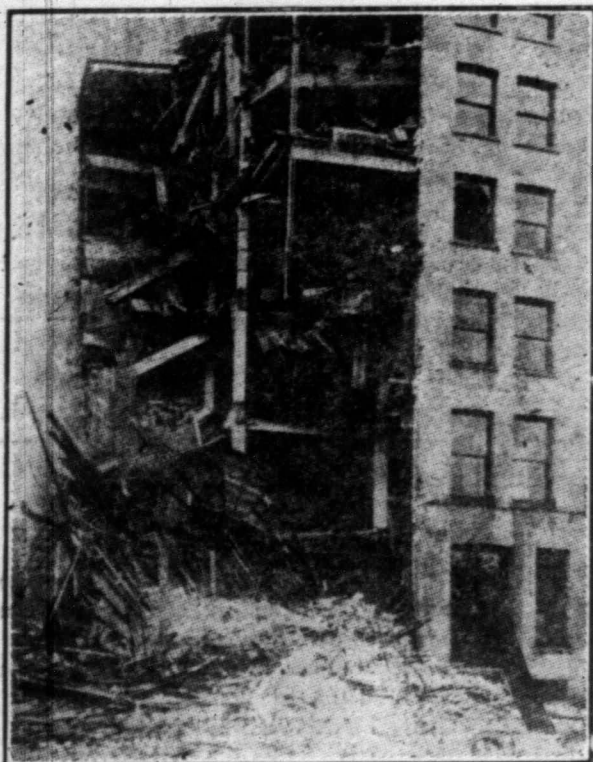
Damage Done by Water Tank.
