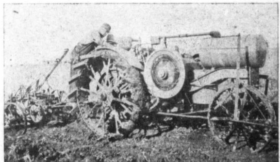
In the thick of a big job—D. W. Heibert, 6th August, 1918
