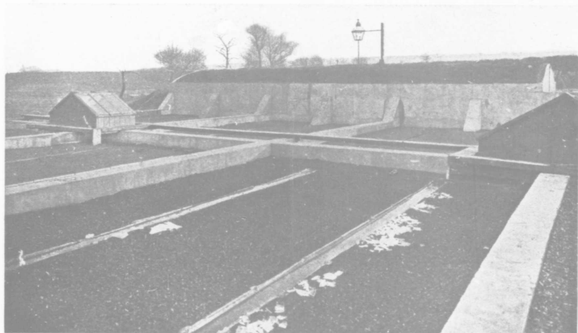
VIEW SHEWING SEPTIC INSTALLATION, MANCHESTER (ENG.) EXPERIMENTS.
