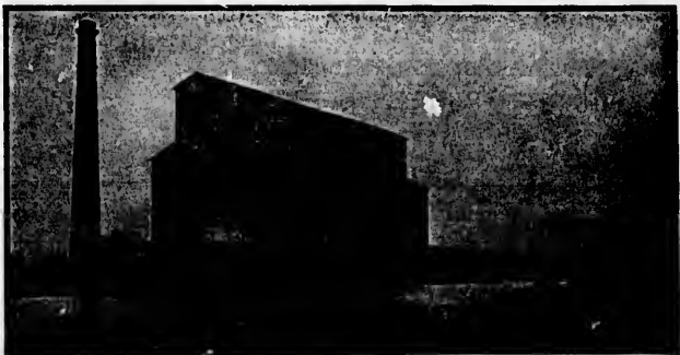
C. F. E. Grain Elevators at Fort William.
