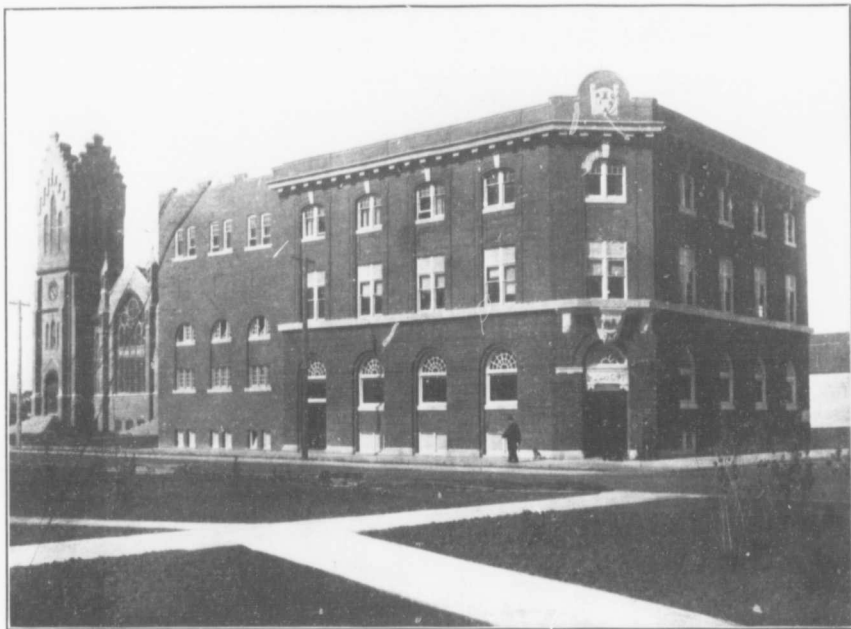
Y.M.C.A. Building, Regina
