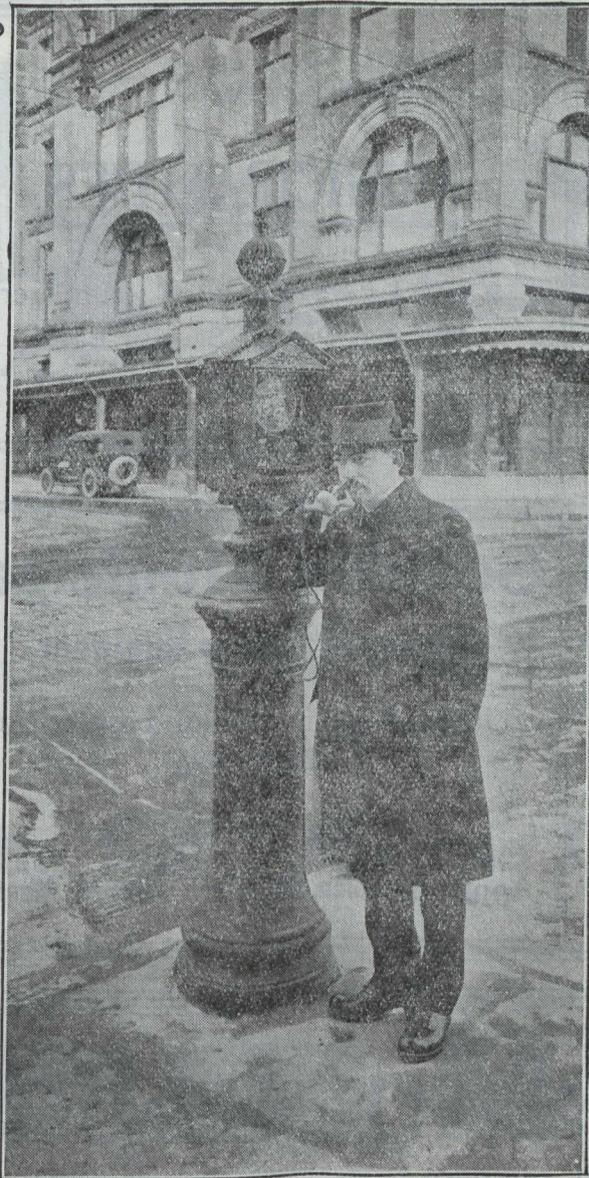
Northern Electric Fire Alarm Post, Outremont, P.Q.—Combining fire alarm and cable terminal box.
