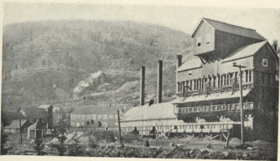
LE ROI MINE POWER PLANT
