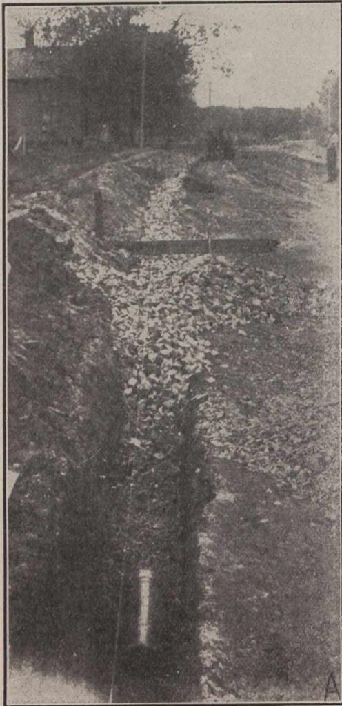
Fig. 3—Tile Under Drain at Side of Road.
