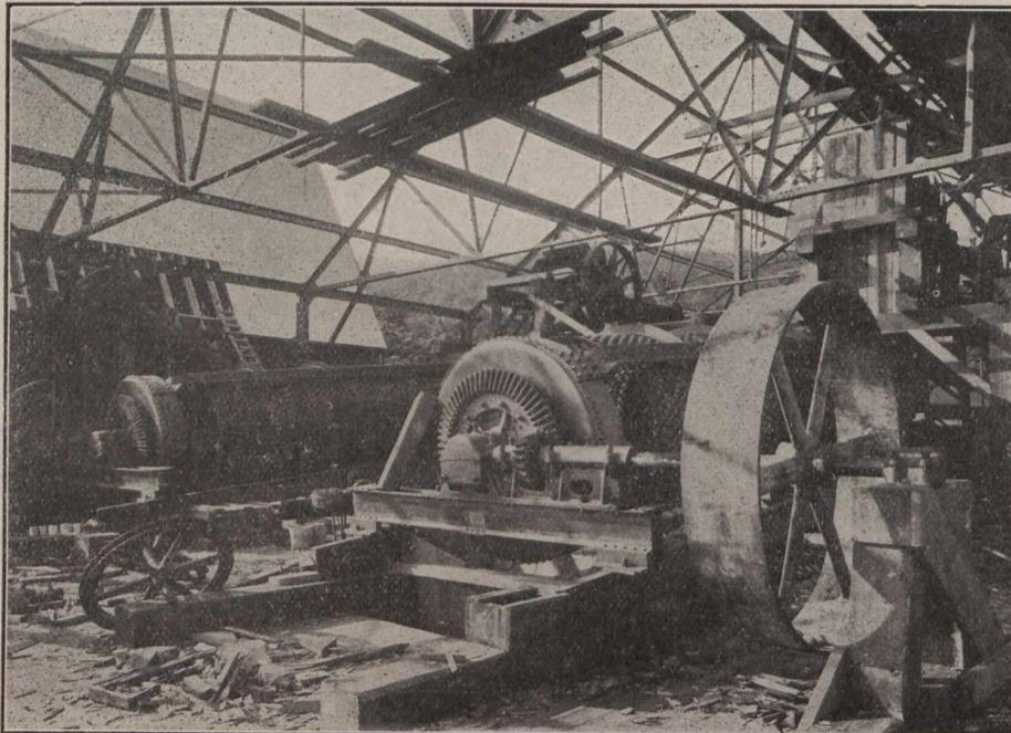
**Taken Under Construction to Show the Chief Screens on the Top Floors of the Crushing Building.**
