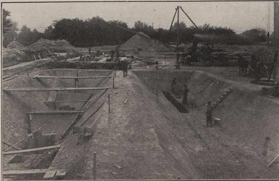
Excavation and commencement of Concreting for Sewage Tanks.
