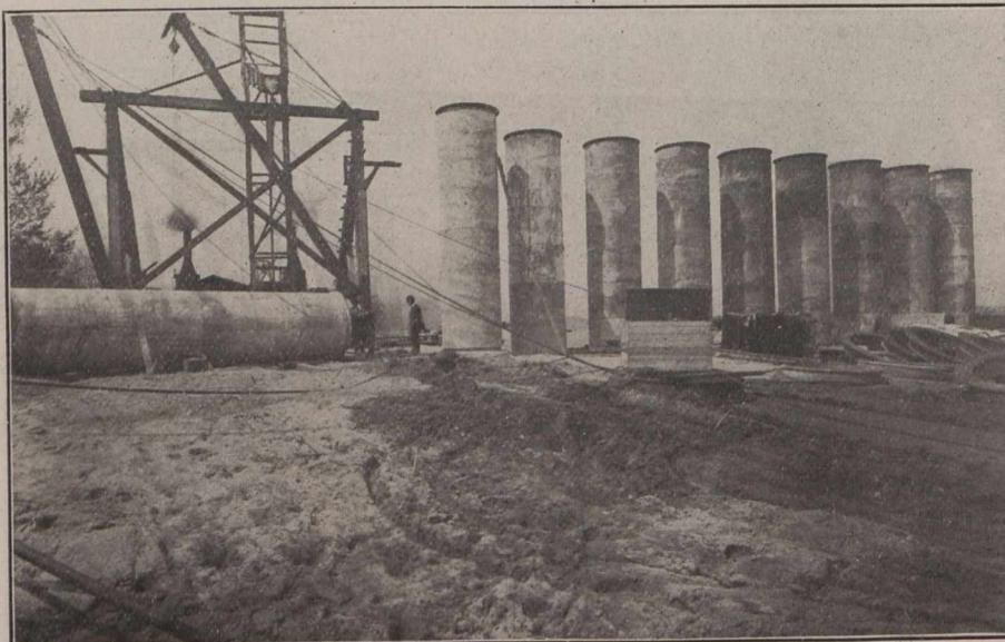
**Reinforced Concrete Pipes (Meriwether patent) for effluent carrier.**
