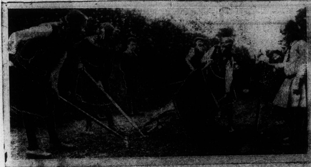
A new roadway in Wiltshire. A little girl "nays" tipping a barrow in a road repairing "gang" in Wiltshire, England, where man help is scarce and the girls have turned in to help to keep things in shape. . .
