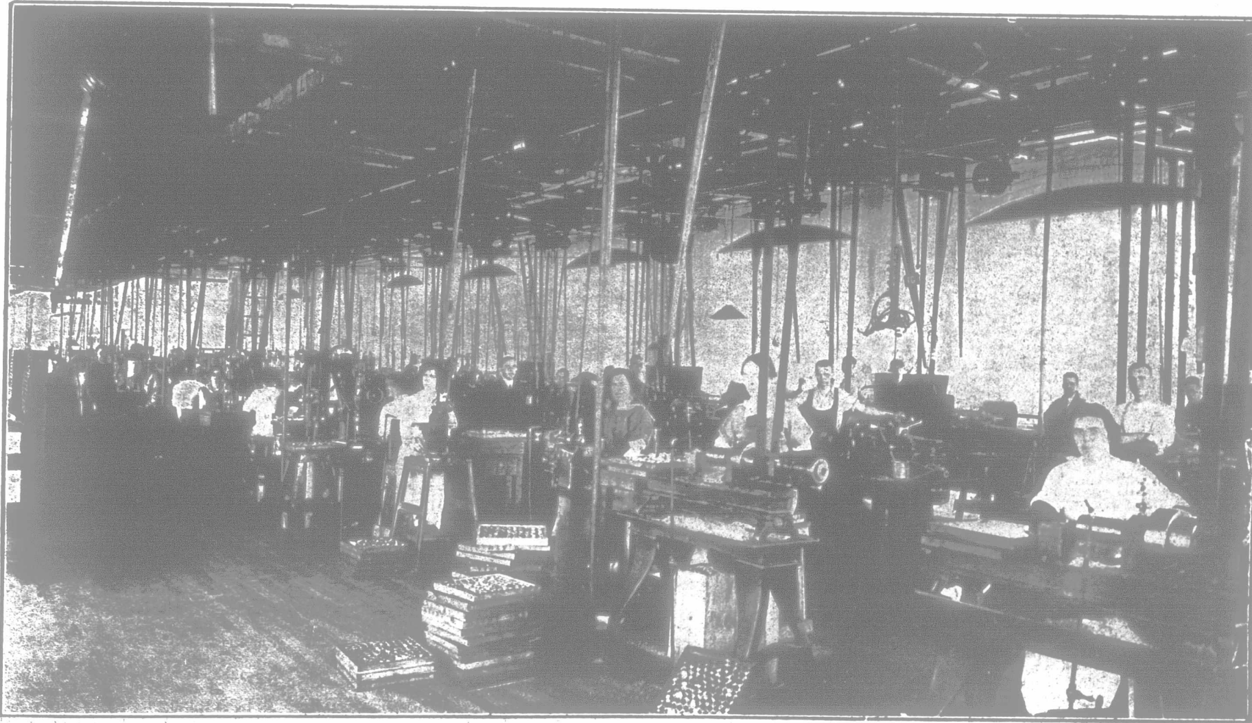
Women Working in Munition Factory, Peterborough, Ont.
